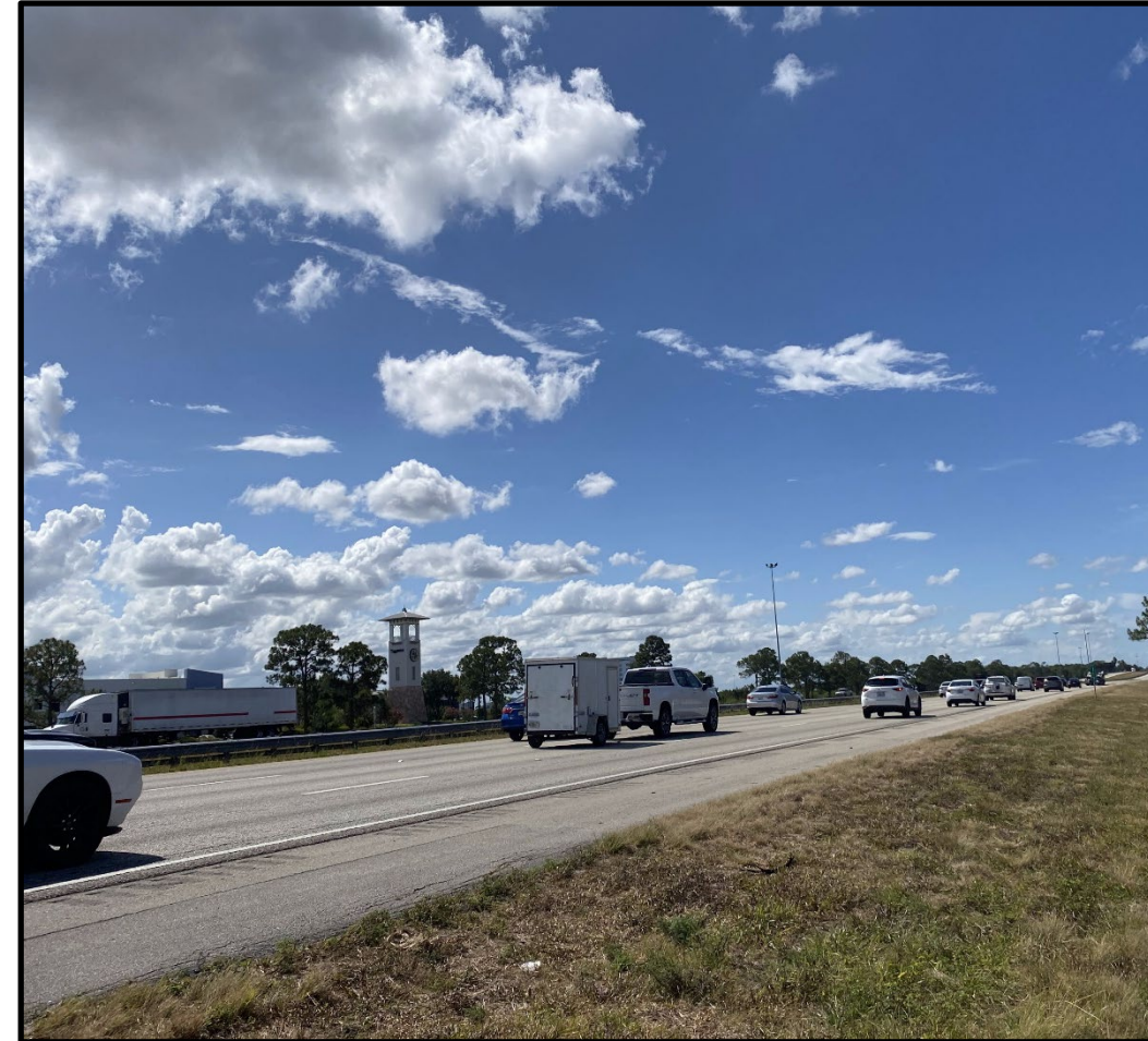
Northbound I-95 (pre-construction)
