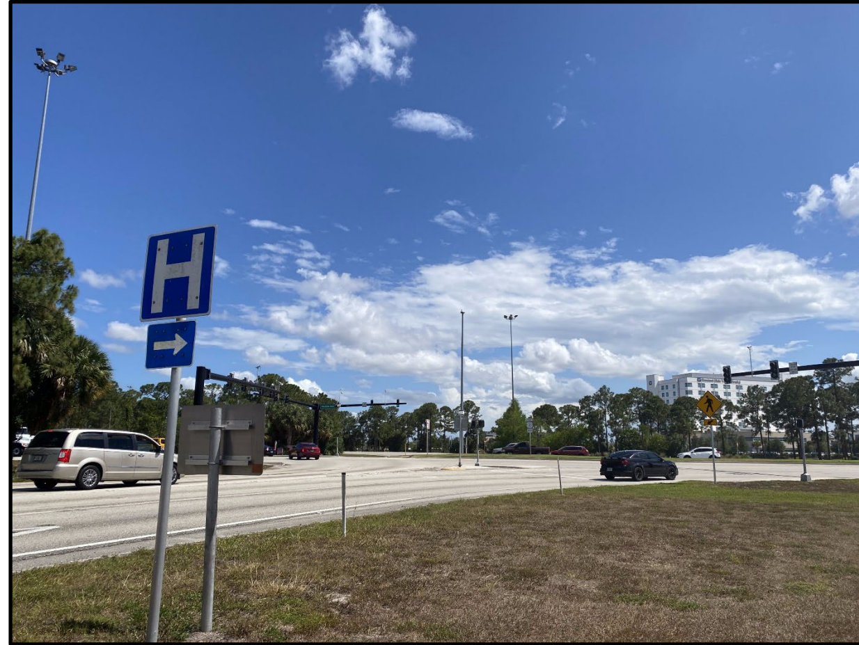
Southbound I-95 off-ramp at Gatlin Boulevard (pre-construction)
