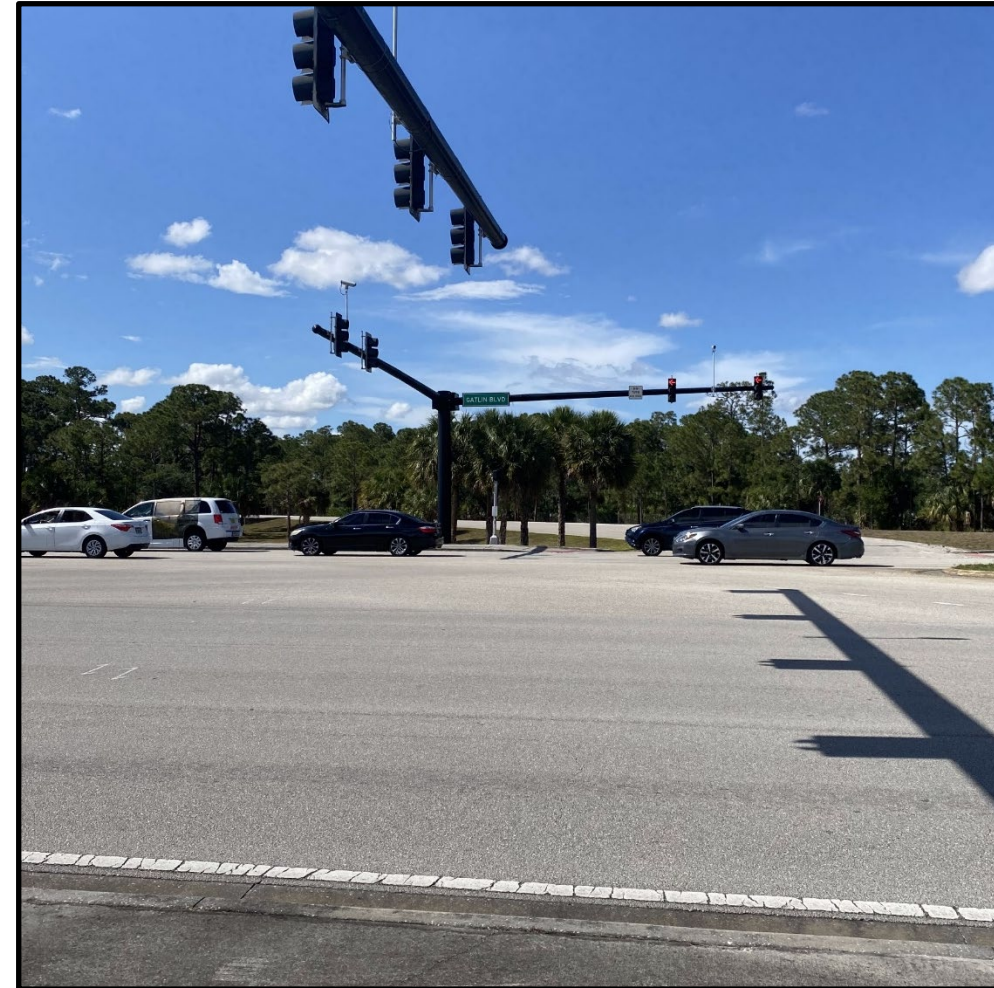
Gatlin Boulevard (pre-construction)
