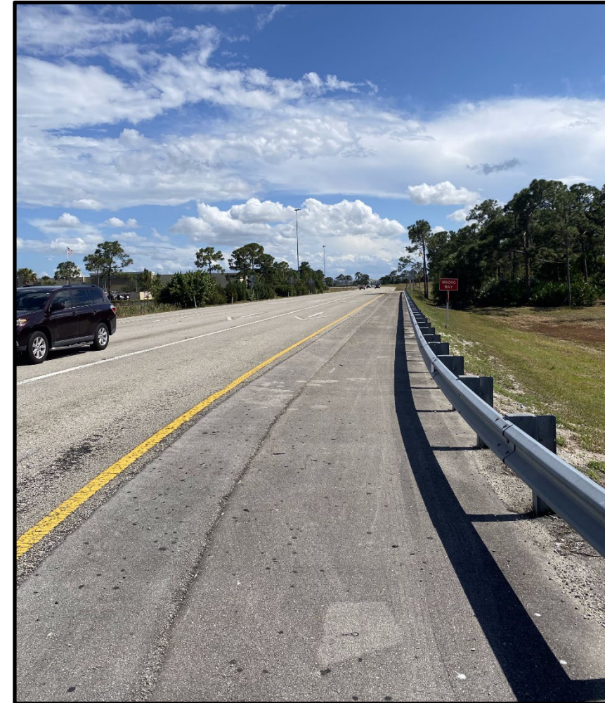
Northbound I-95 off-ramp at Gatlin Boulevard (pre-construction)
