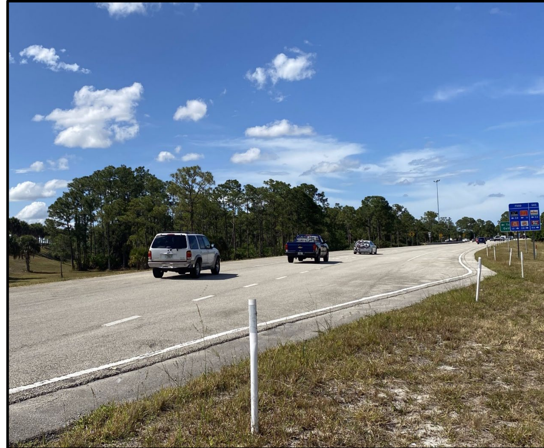
Northbound I-95 off-ramp at Gatlin Boulevard (pre-construction)
