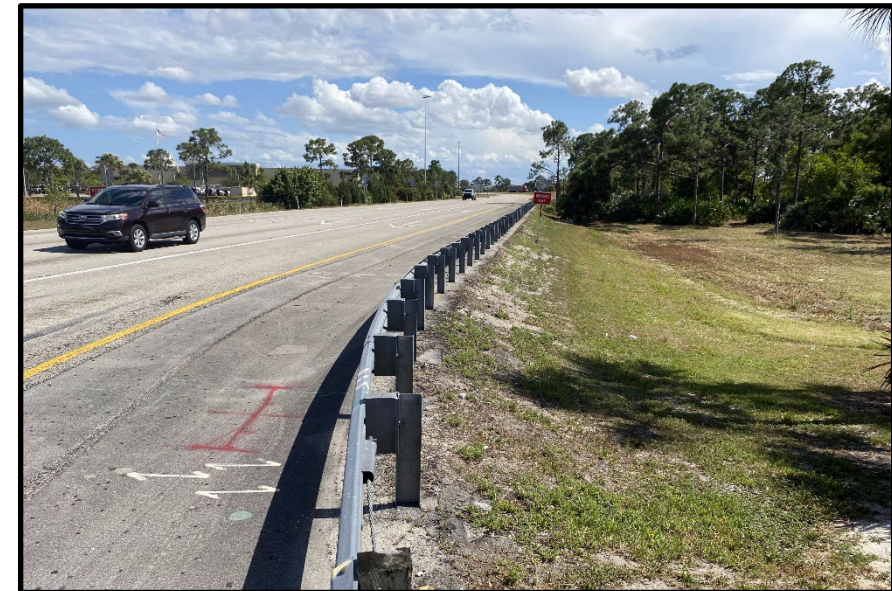
Northbound I-95 off-ramp at Gatlin Boulevard (pre-construction)
